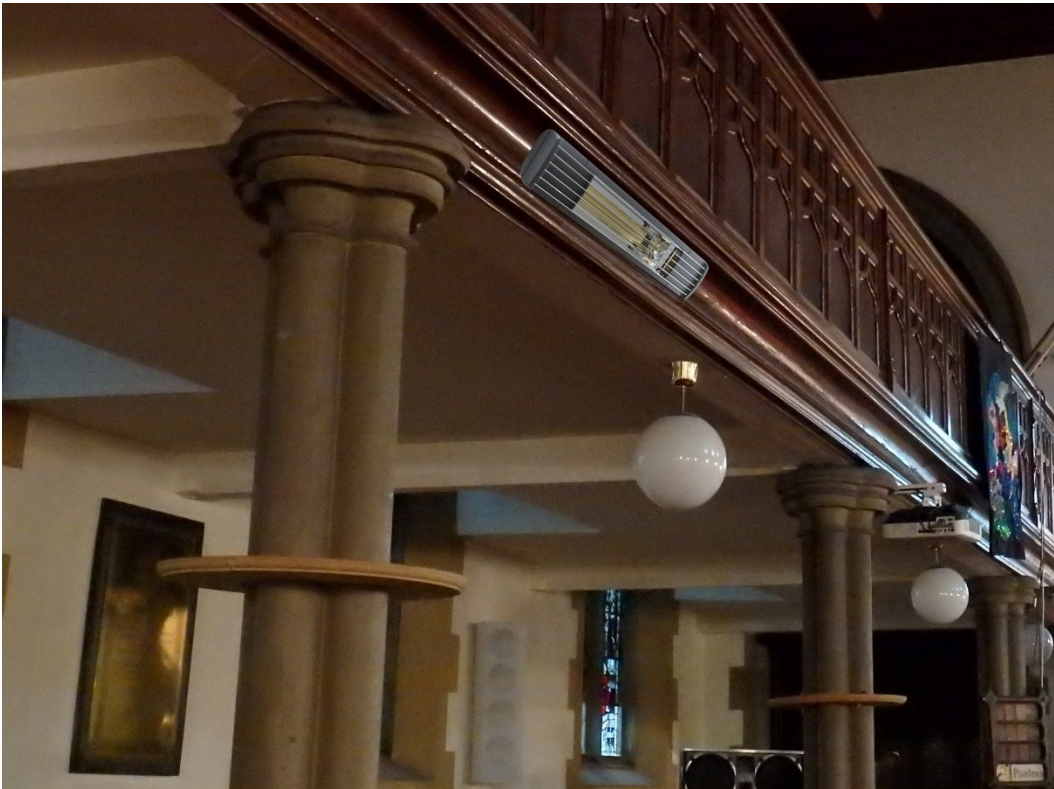
Photograph of north balcony with picture of heater added showing the typical positioning of the heaters in Zone 2 of ARC's diagram. Note that these heaters will be black finish to maximise unobtrusiveness.
